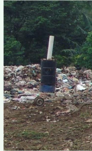
Above: One of the vents in the landfill, giving off less harmful CO 2 and passively sucking air into the pipes for aerobic garbage / leachate breakdown.
